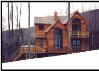
Mountain-Near House 38 Northface
